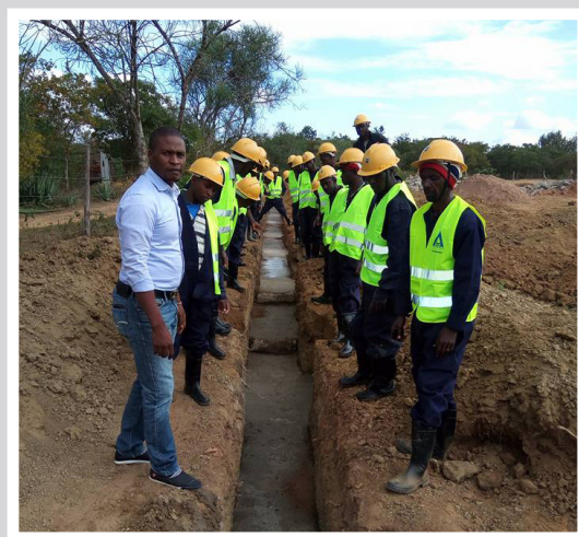
Phase 2: Foundation for classroom blocks laid.
